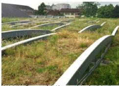
Undulating Green roof that has a variety of soil depths.
